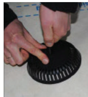
Overdelen presses ned mod undertaget.
